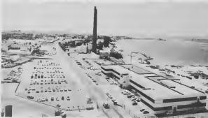
View from top of the PCAR looking east to Serco Colorado.
